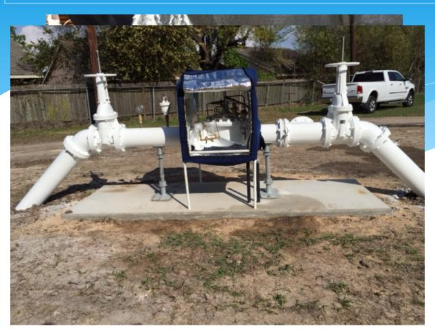
The Freeze Guard TempShield canvas is an excellent reflector of radiant heat to protect the Cla-Val valve from exterior UV rays and internally insulated against freezing. The Freeze Guard TempShield canvas is light weight, strong, puncture and tear resistant. The custom fit allows easy access for all valve maintenance or service. The PVC frame is non-corrosive and built to fit each size CLA-VAL pilot systems.
