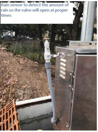
The system is able to 1). open on an upstream and downstream level requirement. 2). open for a rain event .
